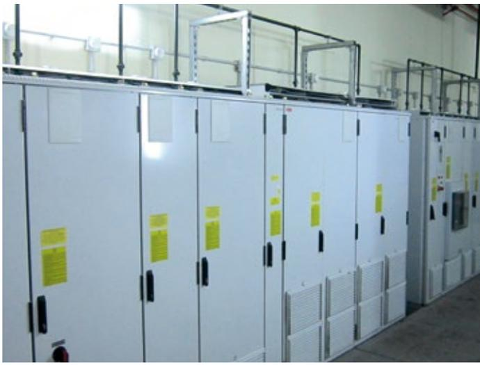
ACS600 drives have been serving the plant's cement production line for more than a decade, being thoroughly maintained to achieve maximum uptime.
