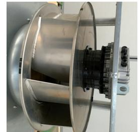
Figure 7: An ECM which is integrated with a VFD (on the right) and the driven fan
