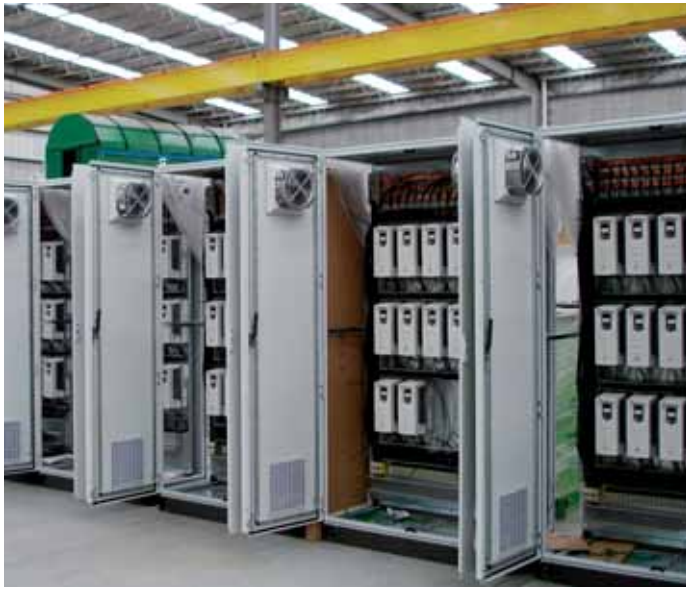
A total of 188 ABB general purpose drives are mounted side by side to save space.
