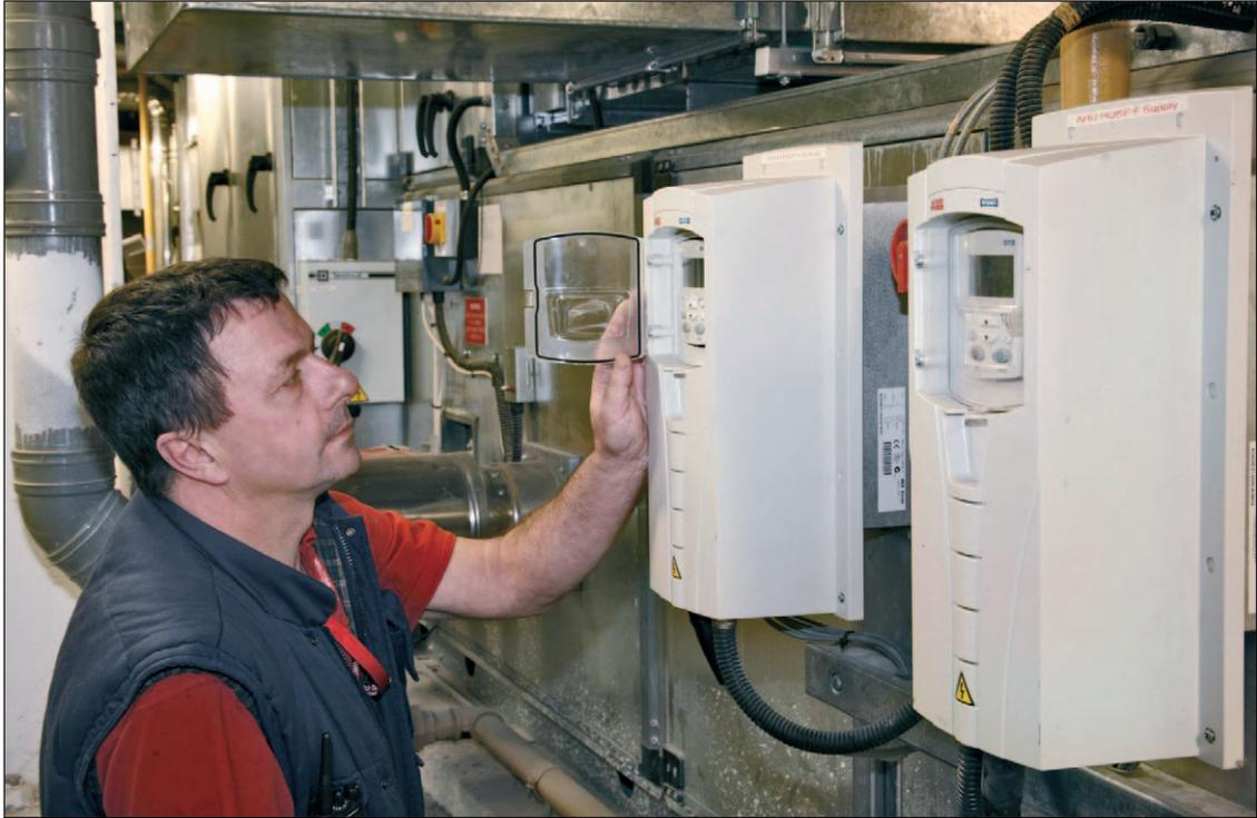
ABB standard drives for HVAC control the fans for the air conditioning system serving the two buildings that comprise the stadium's Quadrant expansion project.
